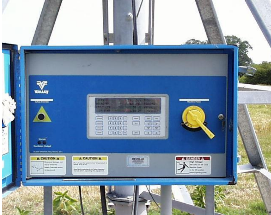
Figure 10-6. Center pivot control panel.
